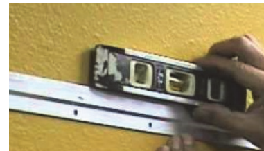
Figure 2. Locating position of the Z-bar bracket.
